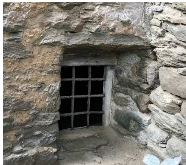
Figura 38: architrave in pietra
